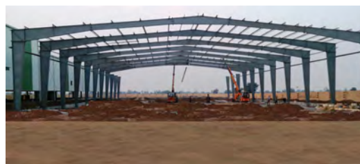
Skeleton Structure Erection
